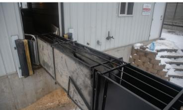
Extension ramp backed up to loading chute
